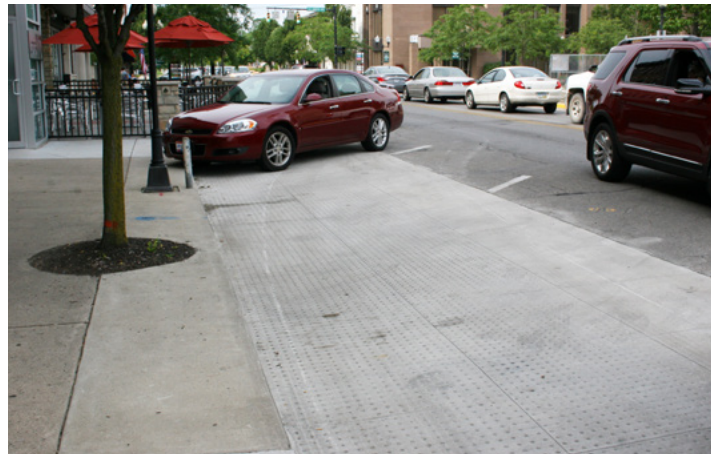
A view of the replicated test strip, which was built with in-kind and cash contributions from people interested in preserving and celebrating the history of the first concrete street in America.
